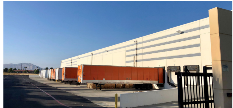
East View of Truck Court
